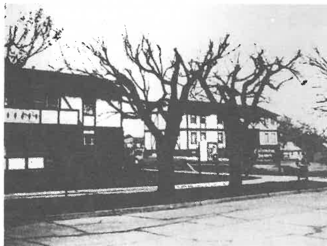
Some of the buildings at Columbia Square today, which won the noted "Landmark Case"
